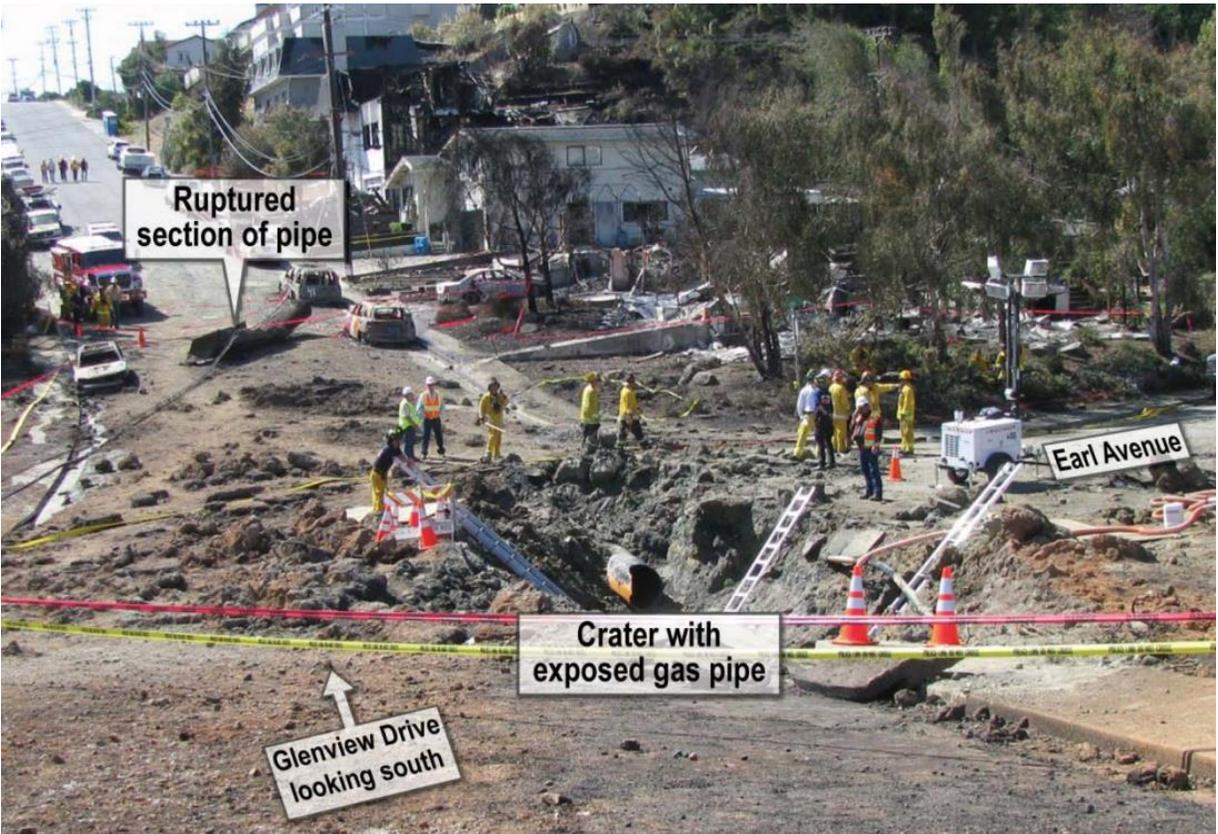
Aftermath of a San Bruno, California gas pipeline explosion that killed 8, destroyed 38 homes, and damaged 70 homes. The "probable cause" of the accident was an "inadequate pipeline integrity management program, which failed to detect and repair or remove the defective pipe section."
